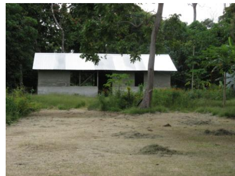
Girls Dormitory (Uncompleted)
