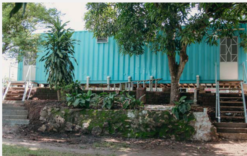
Before and after of the container that has been converted into a shared toilet block . This facility is used by approximately 90 individuals on a daily basis. There are four toilets for males and four for females.
